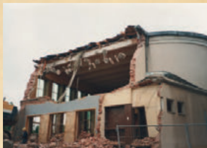
Abriss UT November/Dezember 1999
